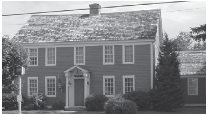
Former Congregational Parsonage - 1306 Boston Post Road 2007 Photo
